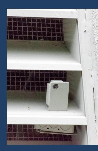
It is Simple Enough To Rig An LED Or Some Sort Of Flashlight To Activate The Photo Cell In This Type Of Setup.
